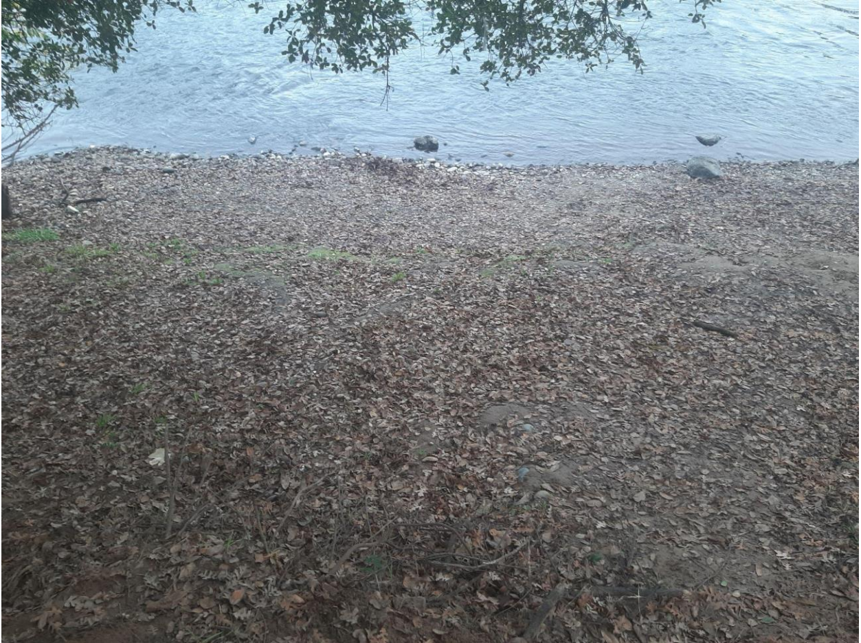
A beach in front of Larchmont Community Park that will be made inaccessible by the Launchable Rock Toe. USACE has not addressed lost beaches due to launchable features.
