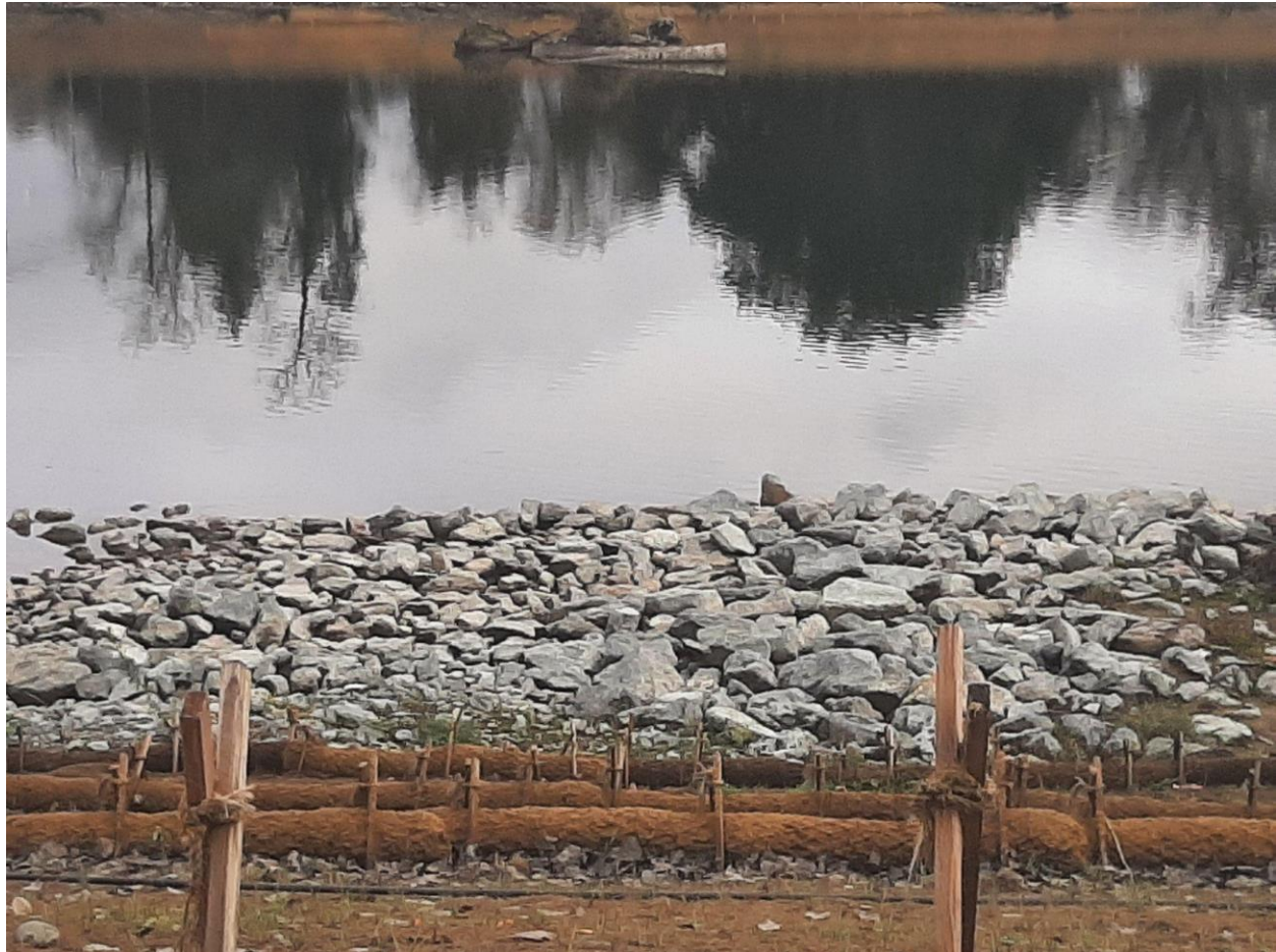
Example of launchable rock toe near Sac State
